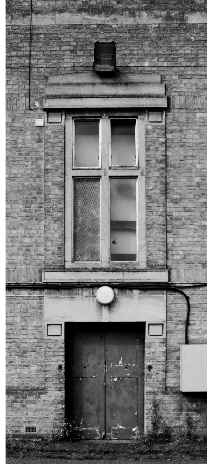
Fig 2: Crash fire door exit on East elevation showing Ketton stone and patent glazing details. The building has meticulous brick and stone detail and restrained Roman decoration with patent glazing largely intact: it is both functional and stylish in concept and execution.
